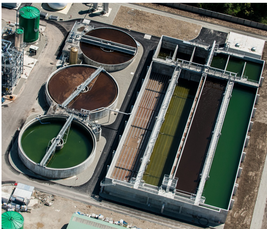
Figure 33: Waste water treatment area
