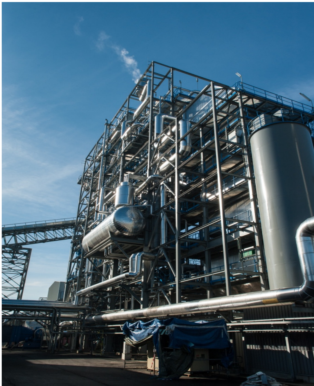
Figure 34: Lignin power plant
