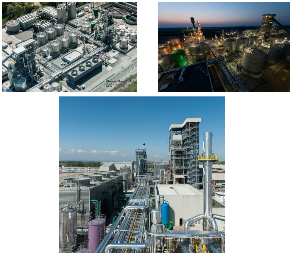
Figure 8: Plant constructed at present day
